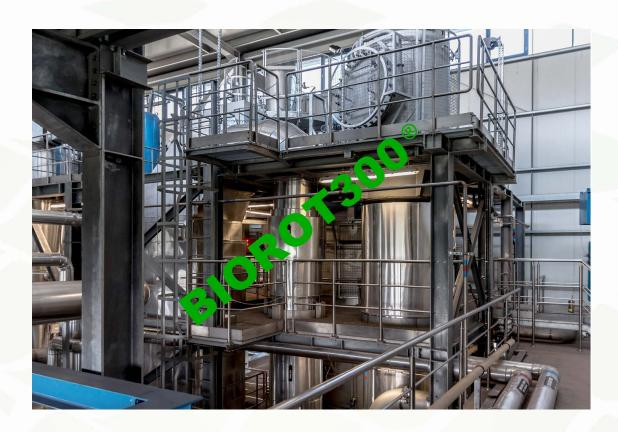
The plant consists of a central rotating main chamber (*patented configuration*) and two fixed parts at the ends: a load front head and a discharge rear head.
