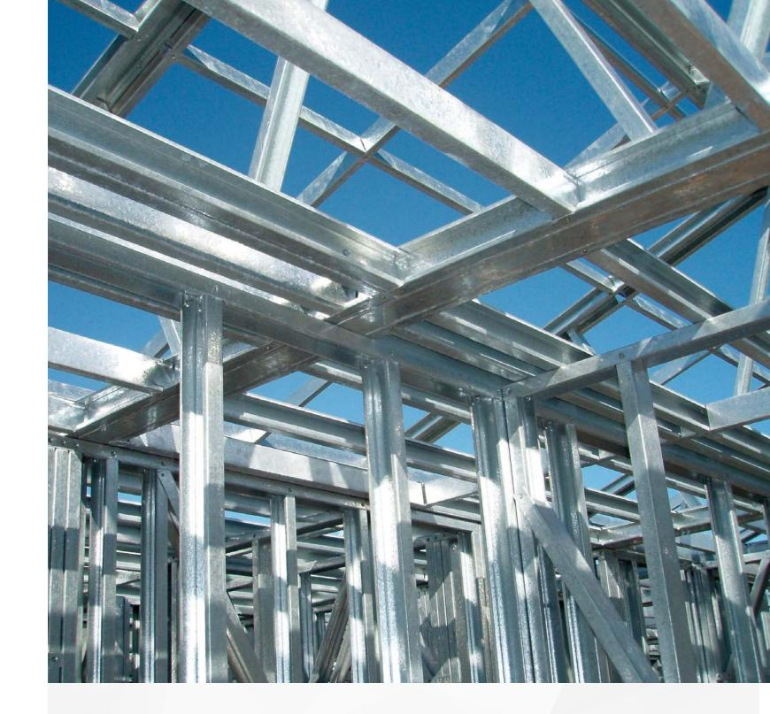
Shorter construction times reduce the hard costs of a project. Buildings using CFS can go up much faster than traditional heavy materials like concrete and masonry. Up to 3 months or more can be shaved off the schedule of a midrise project.
